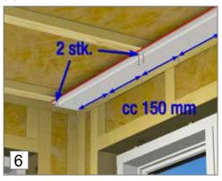
6. Nail spacing is cc 150 mm against wall and double nailing/screwing on each lath.
