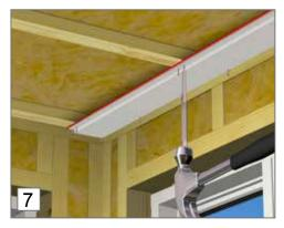
7. To prevent damage to the panel boards, used a punch when nailing the boards.
