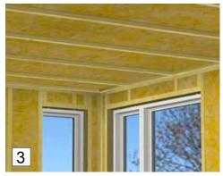
3. Install across electrician's laths/battens spaced at intervals of max. cc 60 cm. When installing on existing screw-mounted ceilings, the panel can be attached independently of laths/battens. For ceilings without screw fastening points for nails/ screws; find the battens and attach the panel to them.
