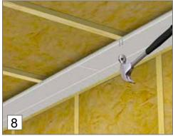
8. The boards must be fixed to electrician's laths or struts and should not be glued.
