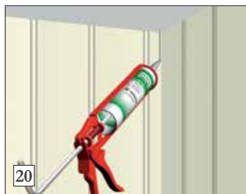
20) We can supply Acrylic Filler in original colours for internal corners if required.
