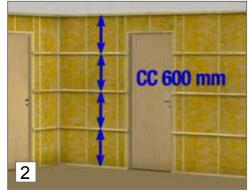
2. If the boards are to be installed longitudinally, the wall must be battened with horizontal battens of max. cc 60 cm.
