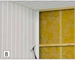
8. The boards must be double-nailed/screwed to each batten.
