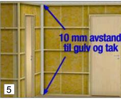
5. Cut first panel board and install 10 mm from floor and ceiling.
