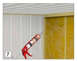
7. First board on a new wall should be glued with Casco superfix or PL 400.
