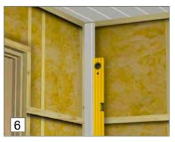
6. Use a spirit level to ensure that the installation starts off right.
