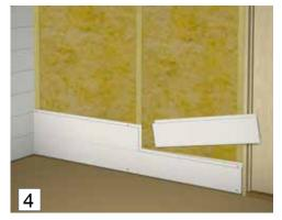
4. Cut the first board to the correct width. When cutting with a circular saw, the painted side must be face down.
